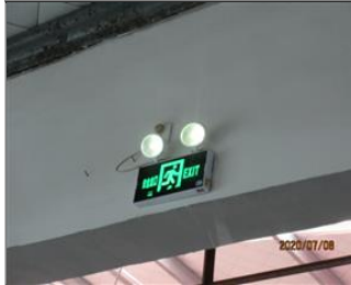
External photo(s) of the production unit(s) testing emergency light.JPG
