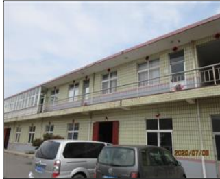
External photo(s) of the production unit(s) office and warehouse building.JPG
